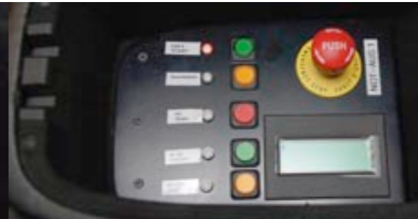
Configuration and monitoring of the systems, installed in the centre console.
